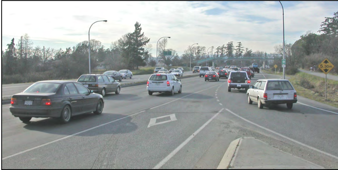
Figure 2 Forced merge, Expressway, 80 kph, right lane is a free RT from the side road
