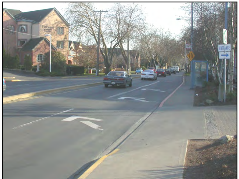
Figure 3a Inadequate Drop Lane design on urban arterial, 50kph
