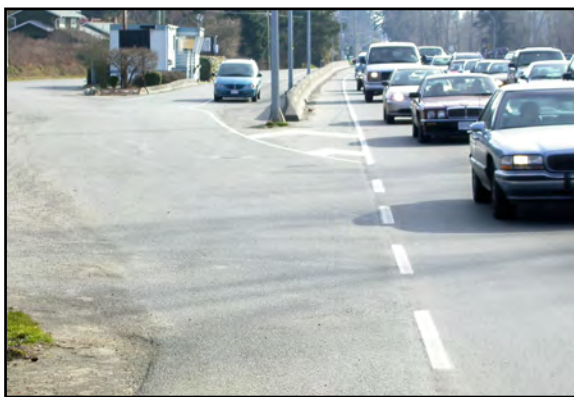
Figure 1 Merge from Highway Pullout, 80kph Expressway, no merge distance.
